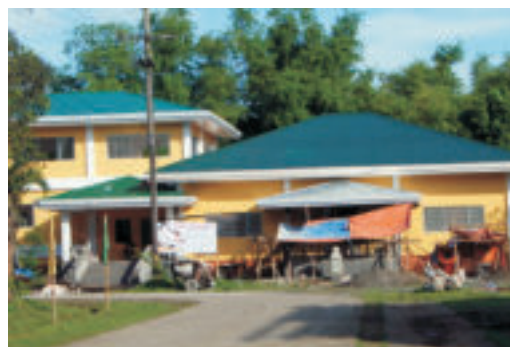
The newly-reconstructed WESVIARC building.
