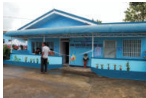
The newly rehabilitated RFRDC Region 5 building inaugurated in August 2008.
